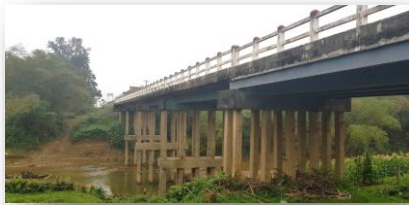
In-situ investigation of the observed bridge
